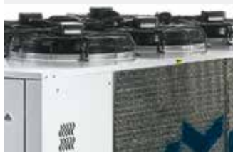
Aeraulically separate sections for the maximum exploitation of free-cooling.
